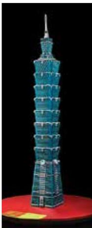
To some people, Taipei 101 looks like a stem of green bamboo. To others it’s a pile of precariously stacked noodle boxes. Able to withstand earthquakes and typhoons, commonplace in Taiwan, this building can sway, literally. A giant pendulum suspended down its center works to counteract external forces, keeping the tower upright.
